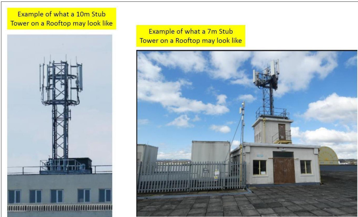
Image 2 - Examples of a 10m & 7m High Stub Tower on a rooftop ( Not to scale and only for reference ).
